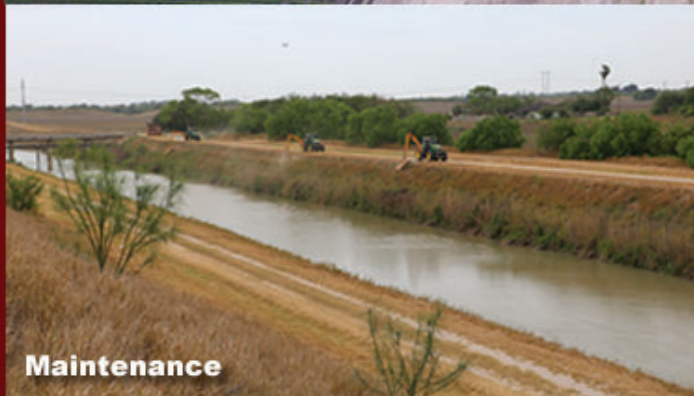
East Lateral Drain
