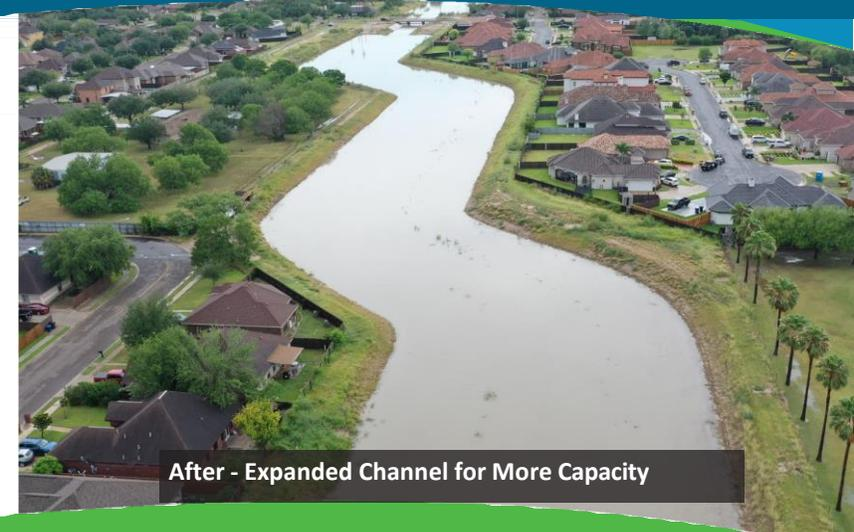
After - Expanded Channel for More Capacity
